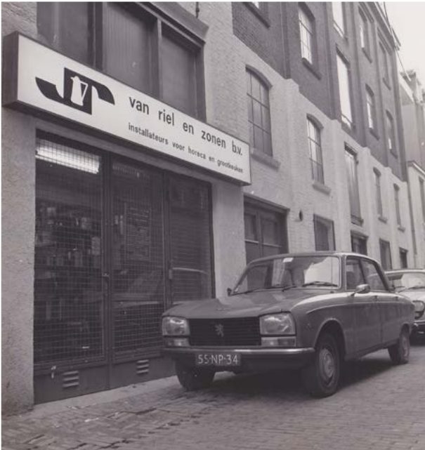
Warehouse in Arnhem in 1976.
